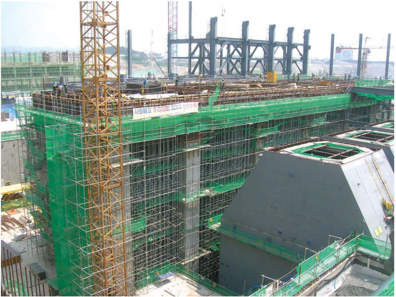
▲ Singori nuclear power plant, Korea. / 신고리원자력발전소
